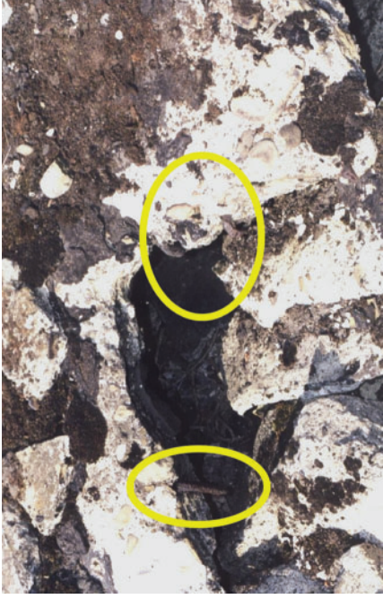
Figure 14. Inwardly bent rebar at north and east edges of second Zyklon hole, partially destroyed in explosion.
