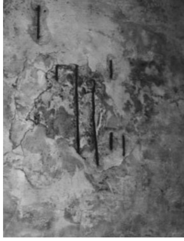
Figure 32b. Sealed ventilation openings in Crematorium I ceiling. It is not known why some rebar crosses opening.
