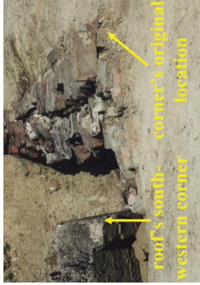
Figure 10a. West-east view of southern edge of Crematorium II gas chamber. Note how roof detached, shifted north, and tipped into hole (for comparison, brick length 23 cm). The shift left the first Zyklon hole farther north relative to first (southernmost) support pillar.
