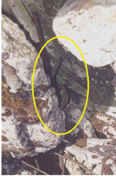
Figure 13. Straight edge and inward-bent rebar on southern side of second Zyklon hole. Such bending could not result from the explosion, which lifted the roof upwards.
