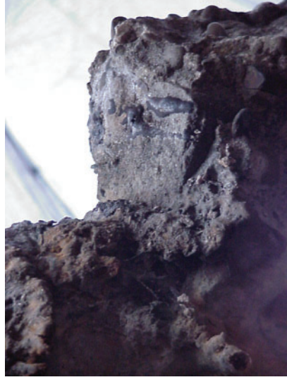
Figure 11b. First (southernmost) Zyklon hole, detail. Taken from below, showing residue of dripping tar. Surviving crawl space approx. three feet here.
