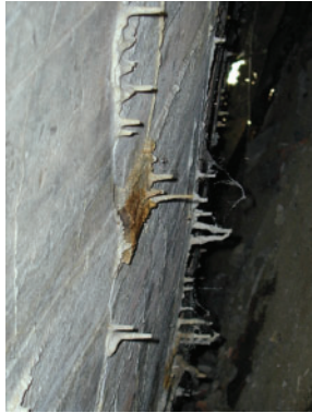
Figures 20a, b, and c. Three of the indentations in the gas chamber ceiling; in 20b (center), rusted rebar just touches inner edge; in 20c (bottom), wood block survives.
