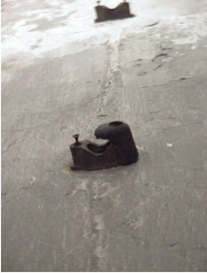
Figure 21. Bakelite supports on central support beam of Crematorium II.
