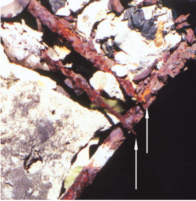
Figure 18b. Rebar stretched to a point at Zyklon hole 1, Crematorium II.
