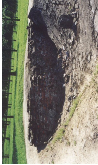
Figure 10b. Northeast-southwest view. Broken top of first support pillar pierces fallen roof.
