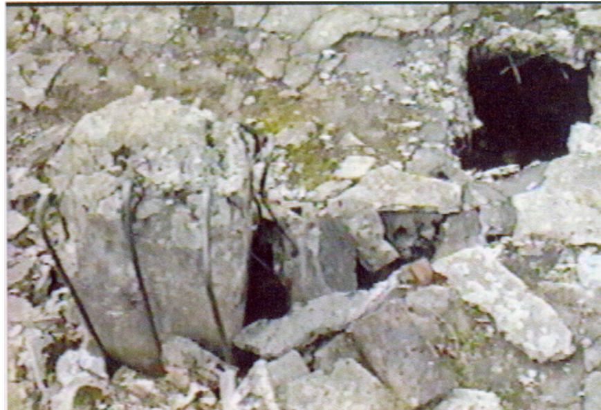
Pillar 1 (left, filling Hole 1) and Hole 2 (right). Note the large wide crack between the two. [View: from the east]
