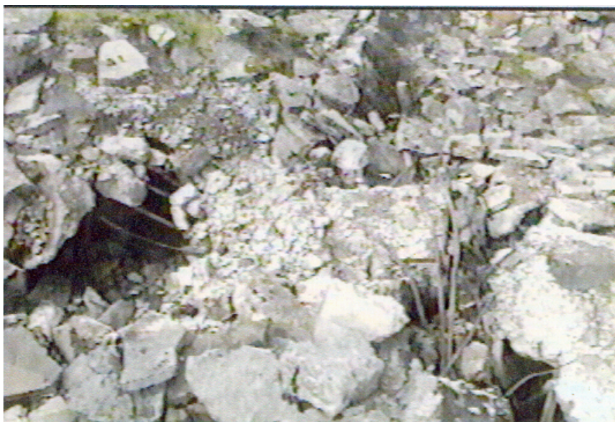
Hole 8, on left with rebar remnants of the central roof column visible immediately above. To the right, the shattered roof around the central roof column. [View: from the east]
